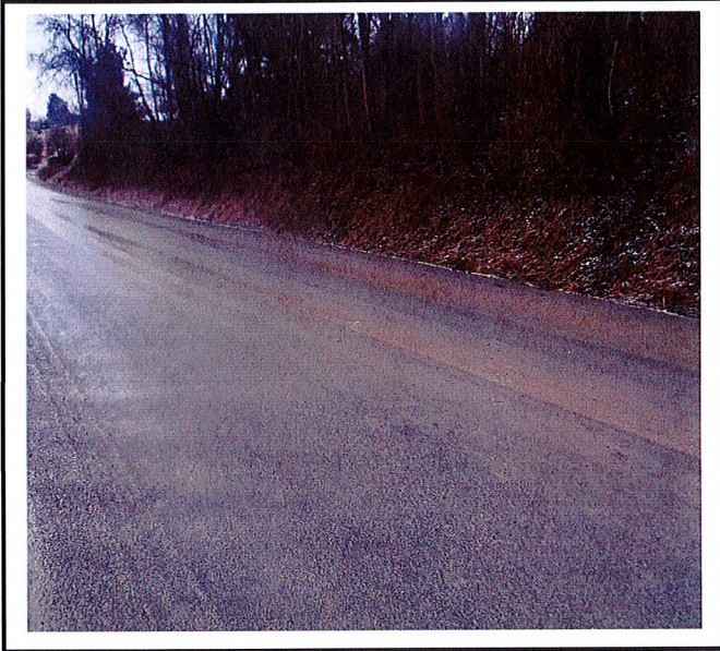
Mud tracked onto Watercure Hill Road.
