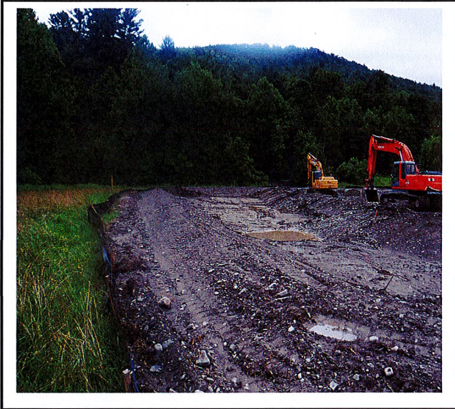
Stormwater basin under construction.
