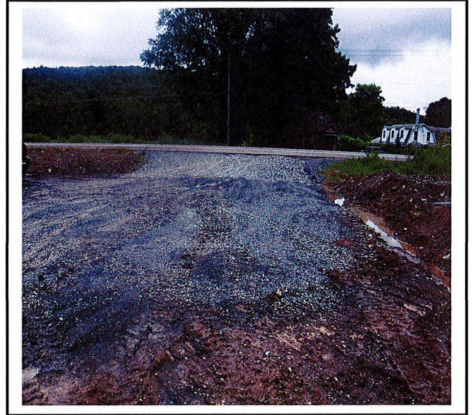
Construction entrance installed.
