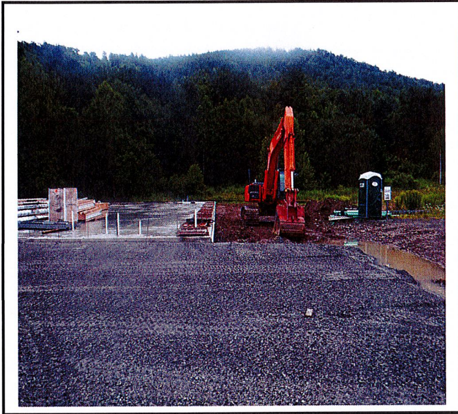
Earth work continues around building footprint.
