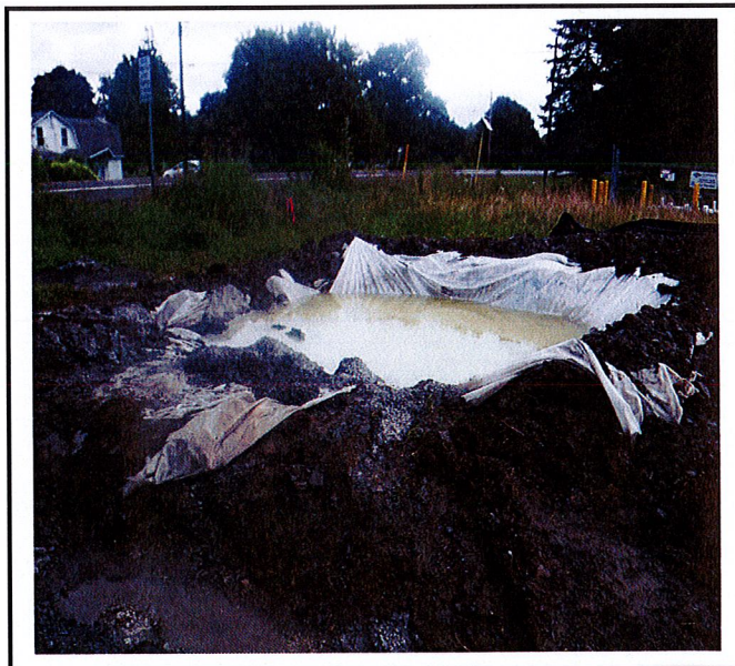
Concrete washout is near capacity.
