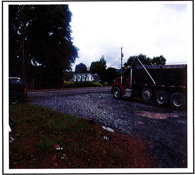
Construction entrance in working order.
