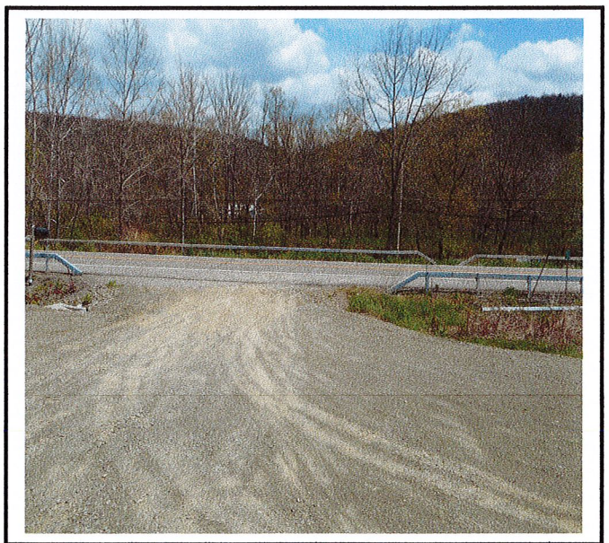
Construction Entrance will need to be re-established once work begins again.
