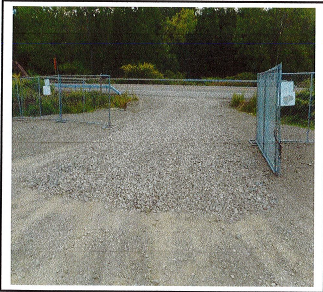
Construction entrance looks good.
