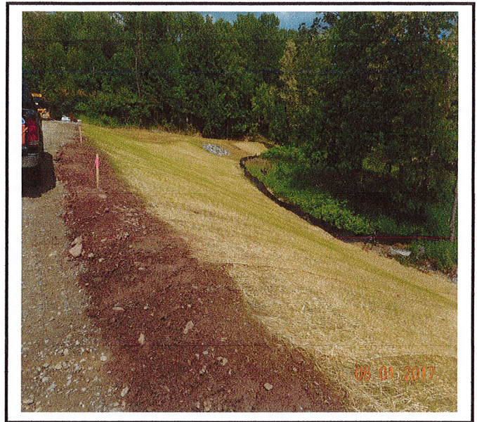
Erosion control blankets have been installed and vegetation is growing.
