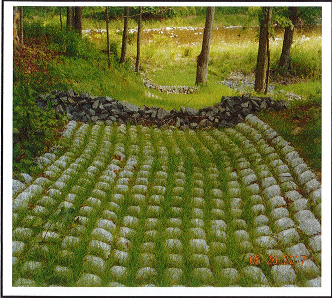
Reinforced slope protection installed.
