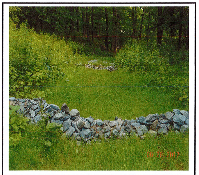
Swale intercepting runoff from Berwick Turnpike.
