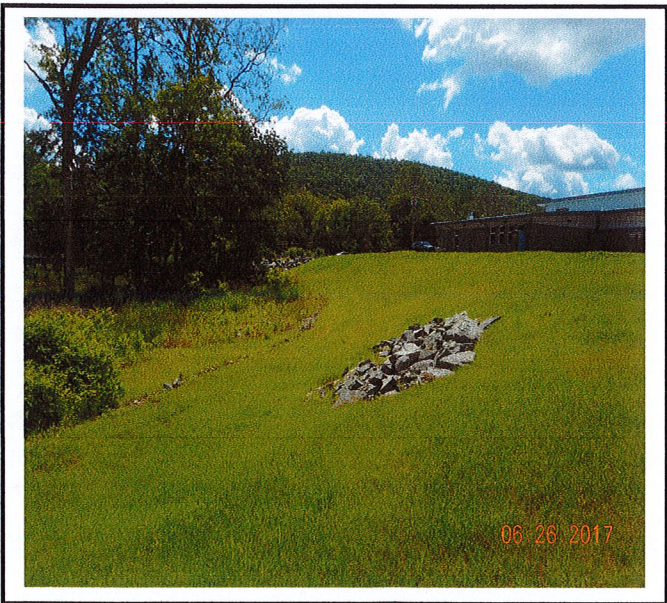
Slopes along Bentley Creek stabilized.
