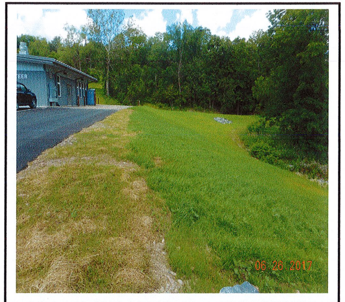
Slopes are well vegetated.
