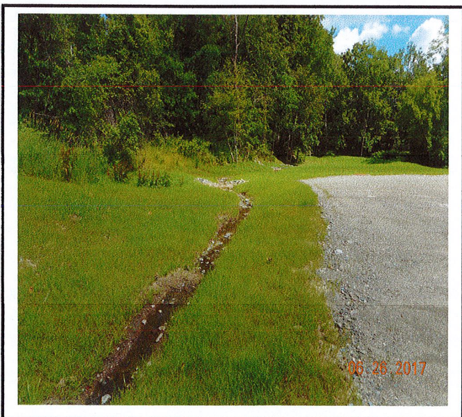
Swale running on south side of parking lot.
