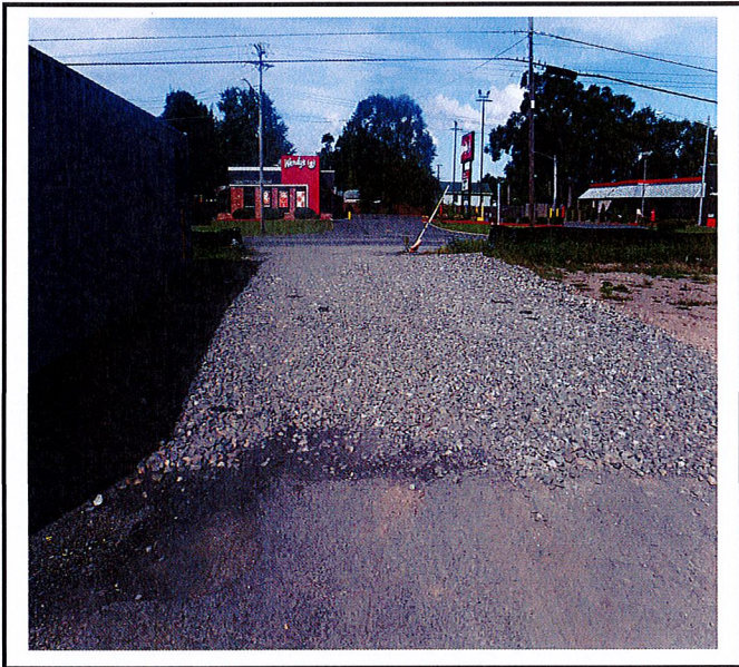
Construction entrance in working condition.
