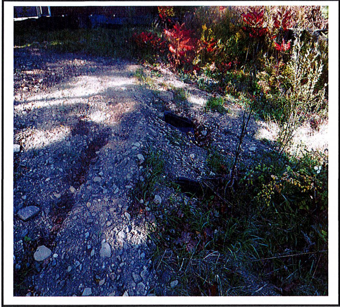
Outlet pipe has been installed into the stormwater pond.
