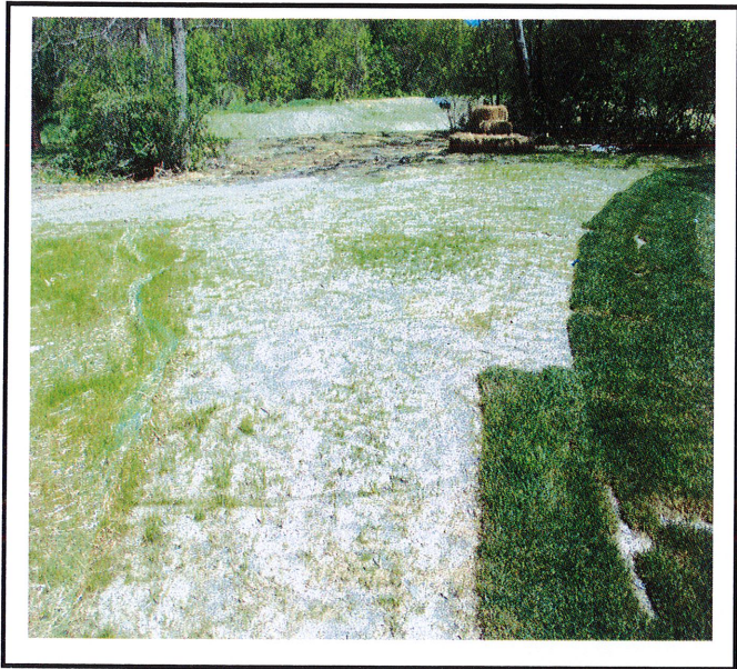
Soil needs to be stabilized to 80% cover. This area is compacted and may need to be scarified to get grass to grow.
