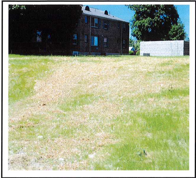
All disturbed soil has been stabilized.
