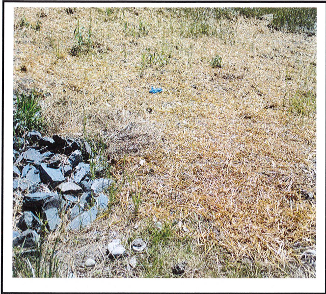
Major erosion spot has been repaired.
