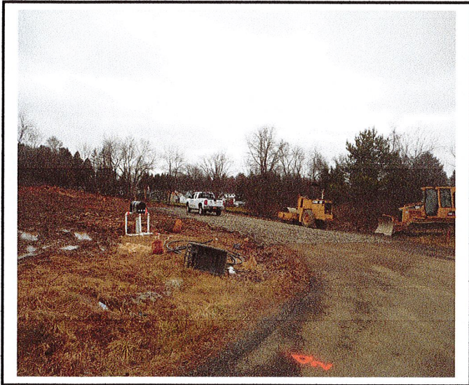
Construction entrance is installed.
