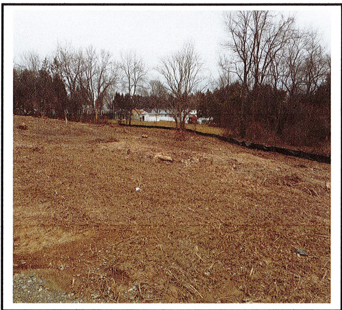
Silt fence along south end of property.
