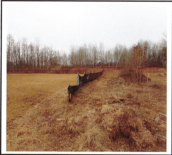
Silt fence has been installed.
