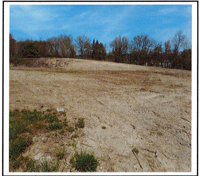
Bare soil has been idle for over 14 days and requires stabilization.
