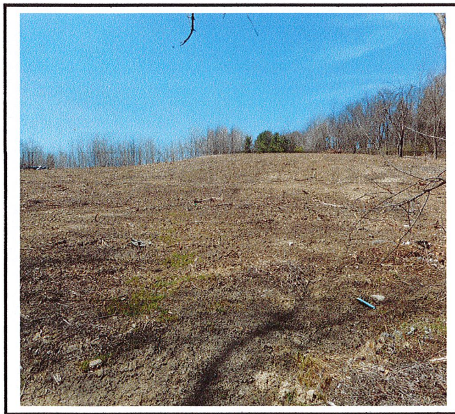
Bare soil areas require stabilization.
