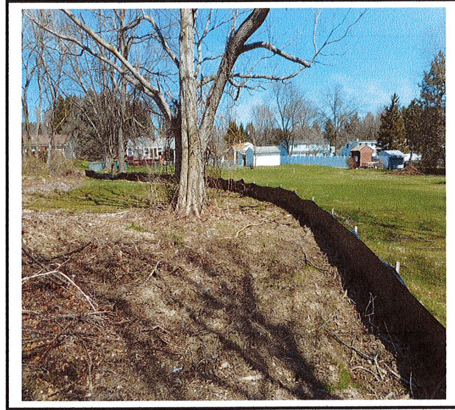
Silt Fence is in good shape.
