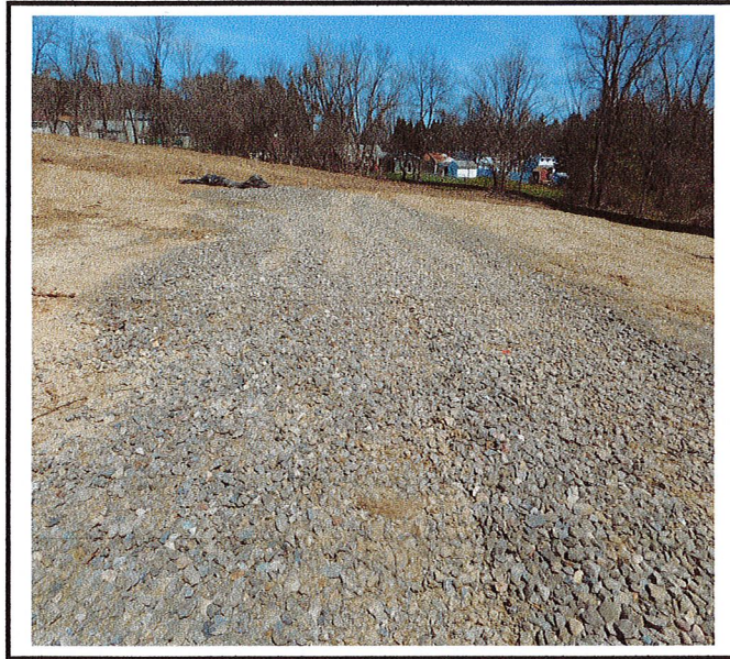
Construction Entrance has been installed.
