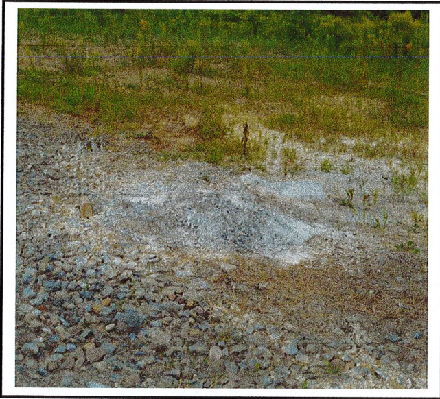
Concrete from neighboring project site was washed onto ground at this site.
