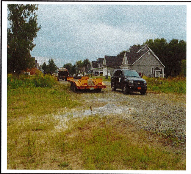
Concrete from neighboring project site was washed onto ground at this site.
