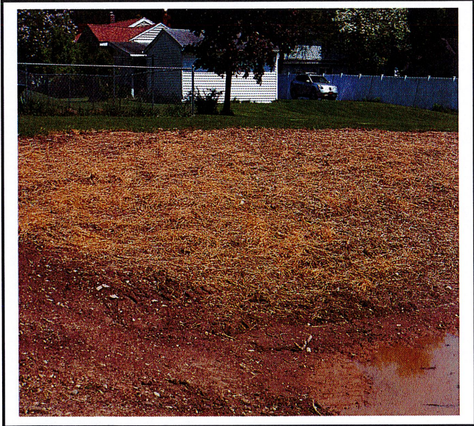
Mulch rates on side slopes does not meet the 2 tons per acre standard.
