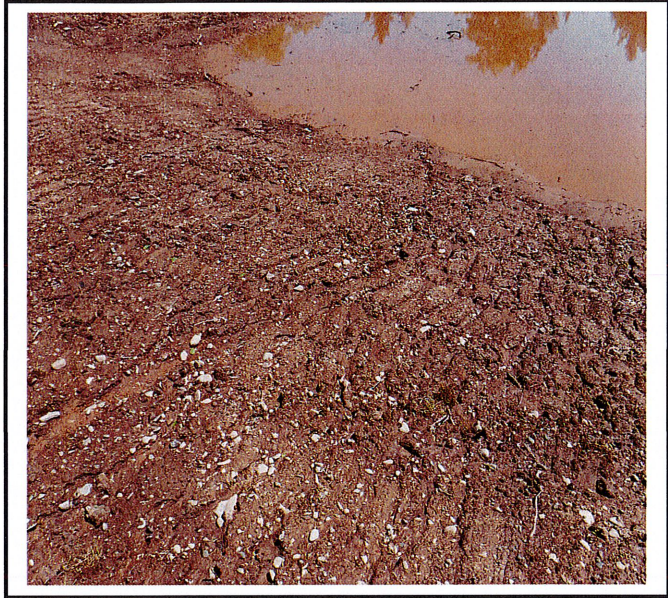
Erosion from heavy rain on the side slopes of the stormwater basin forebay.
