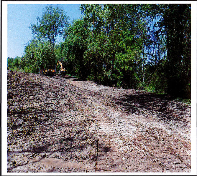
Drainage swale along north end of property being constructed.
