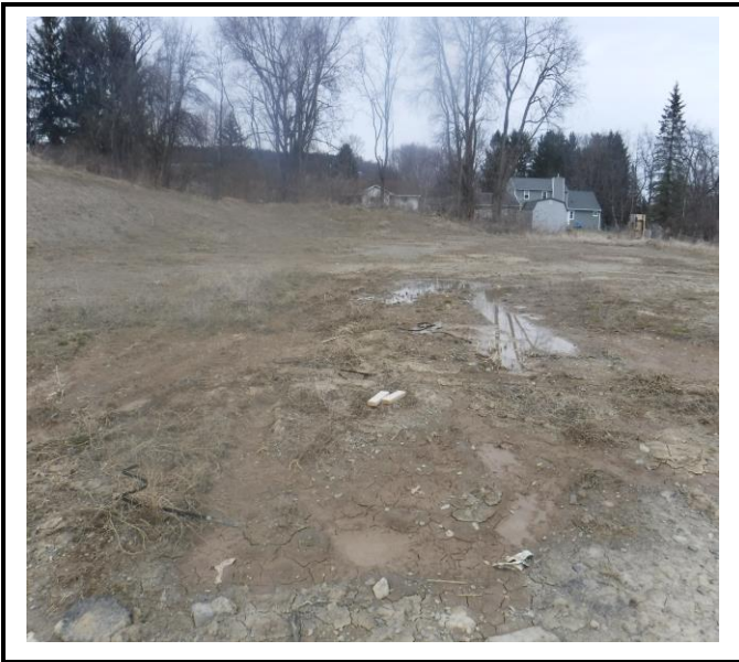
Driving and working in areas that are beyond the limits of disturbance of the 2 lots approved for work.
