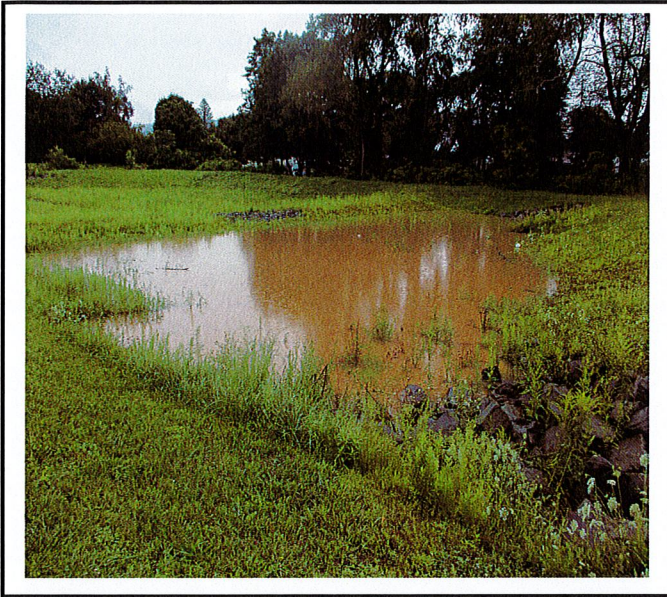
Forebay of infiltration basin is filled with muddy water.
