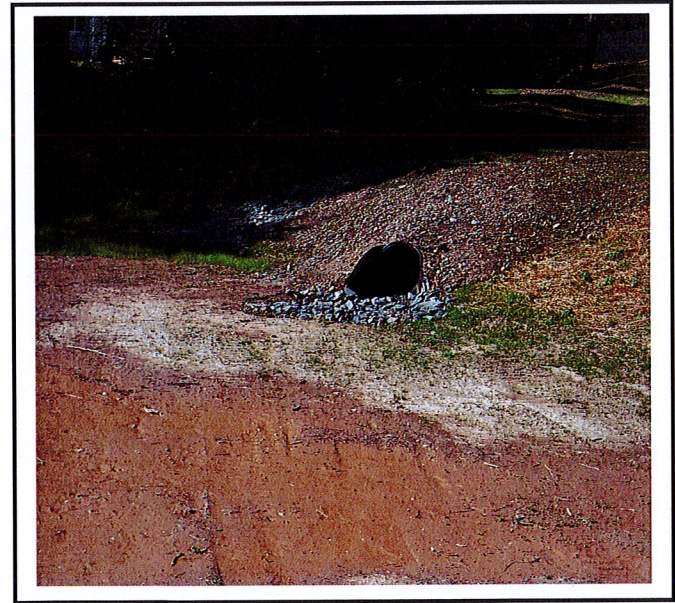
Swale inlet and storm sewer inlet on south side of forebay.
