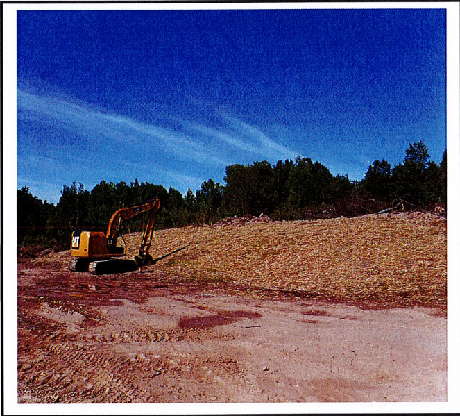
Slopes on west end of phase 1 have been properly stabilized.
