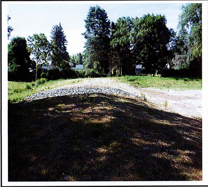
Emergency Spillway in stormwater retention basin.
