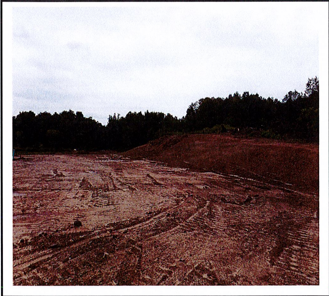
Graded areas around buildings 7,8, and 9.
