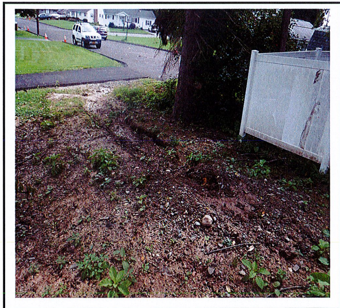
10' utility easement needs to be stabilized.
