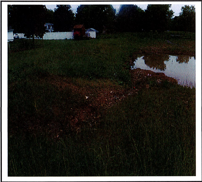
Erosion in drainage swale down to stormwater basin. This erosion needs to be repaired and all of the sediment in forebay needs to be removed.
