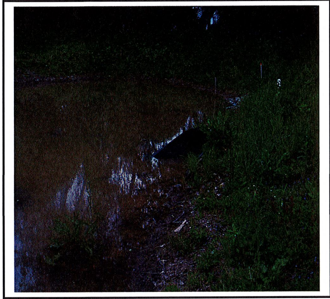
Rock outlet protection not installed on the end of this pipe.
