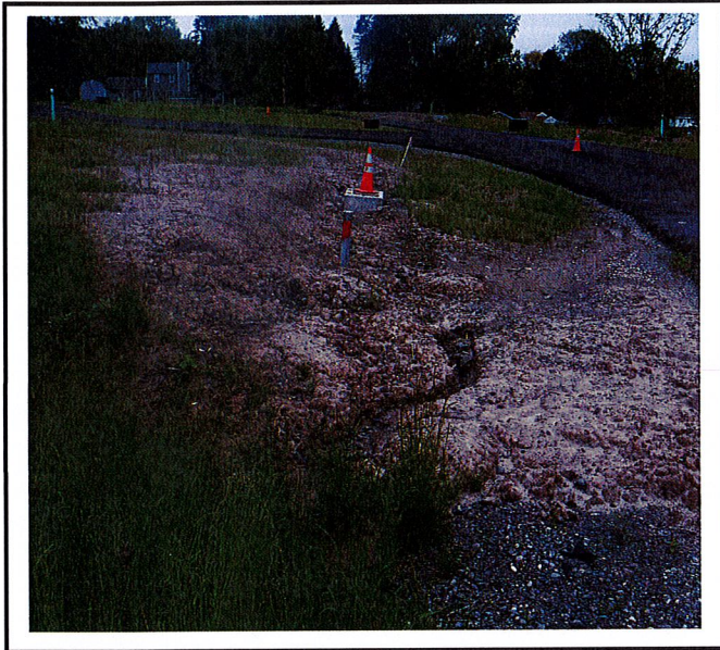
Erosion is occurring in all areas not properly stabilized.
