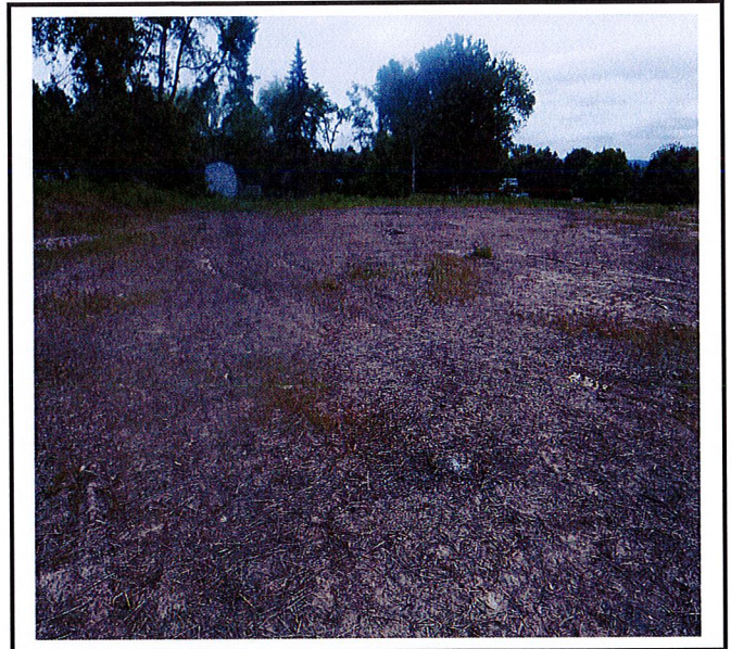
Many areas that were stabilized last fall are not growing grass and mulch is no longer there. These areas need to be re-stabilized.
