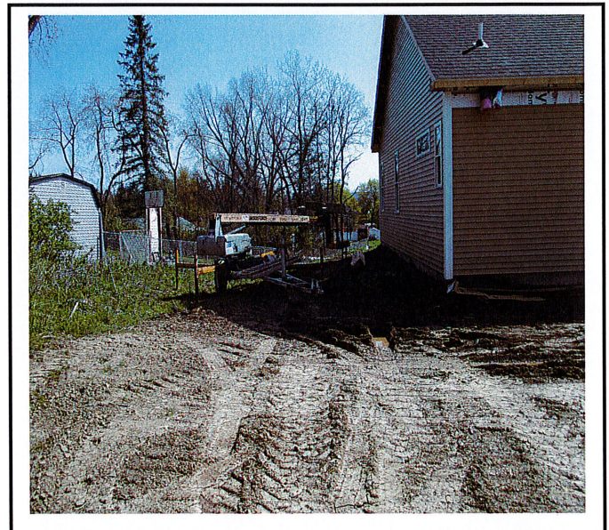
Equipment partially parked in stormwater drainage channel.
