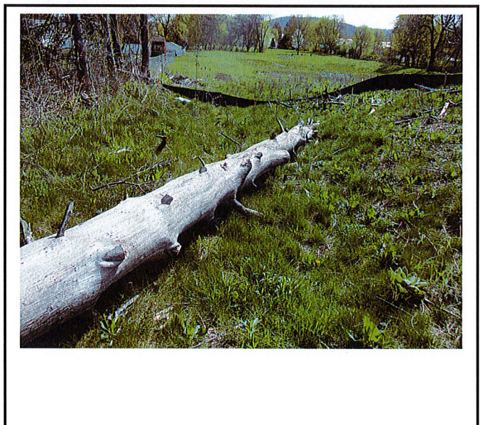
Silt fence across ditch (photo from April 2021) that need to be removed from drainage swale.
