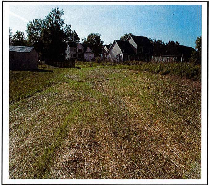
Stormwater drainage swale behind Lot 9 has been constructed and stabilized.
