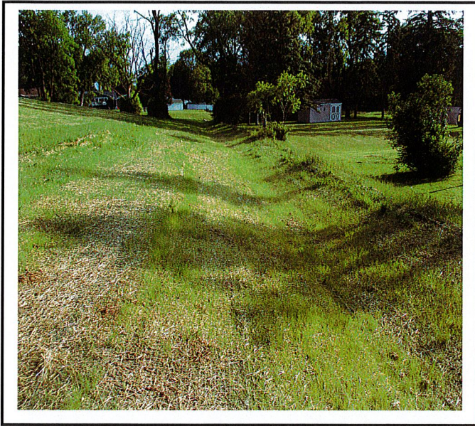
Stormwater drainage swale along Lot 1, 2, and 3 reconstruction is complete.
