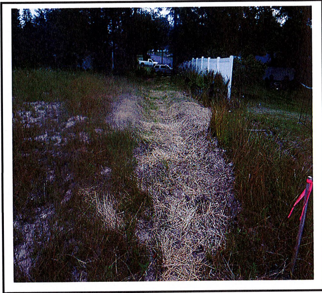
Drainage swale along the perimeter of property.
