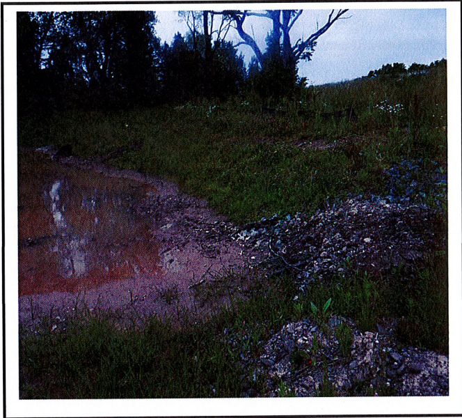
Sediment eroded into the pond will need to be excavated when the entire project is finished or when 50% capacity is filled with sediment.
