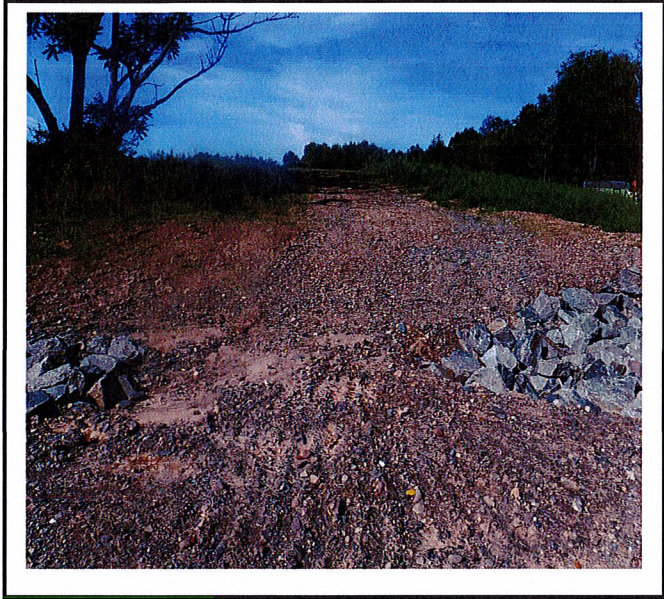
Graded area on Lot #4 leading down to stormwater basin is showing signs of erosion. Stabilization is required.
