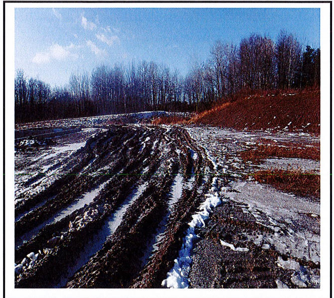
Construction vehicles are driving outside of lots under construction and tracking mud everywhere.
