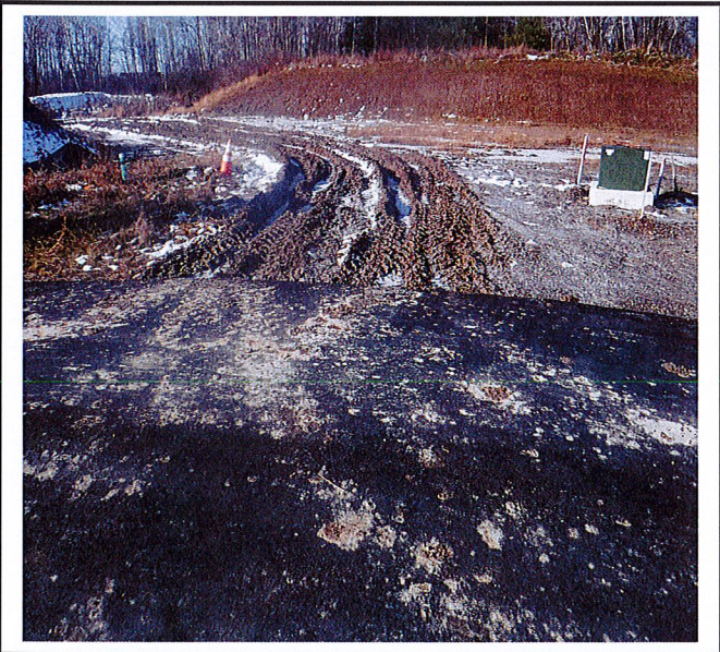
Construction vehicles are driving outside of lots under construction and tracking mud everywhere.
