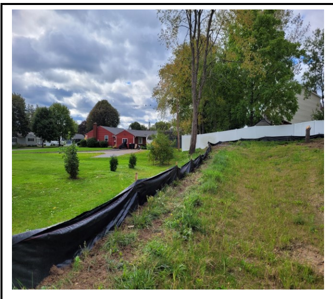
Silt fence along property line.
