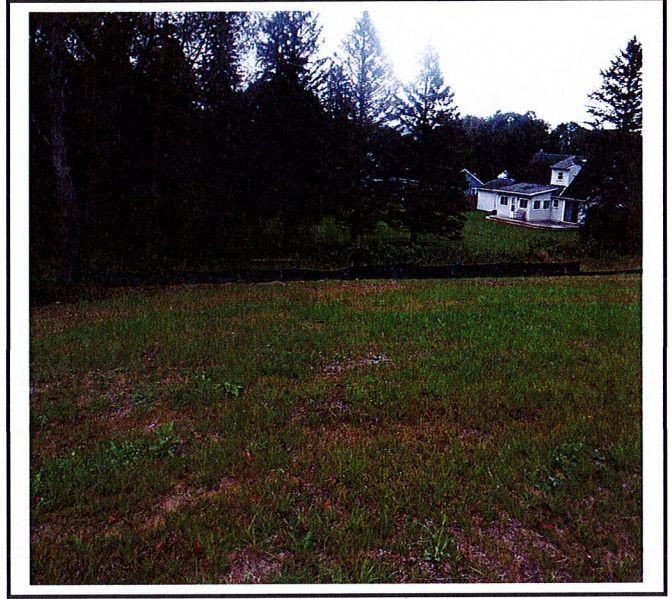
Silt fence has been repaired.
