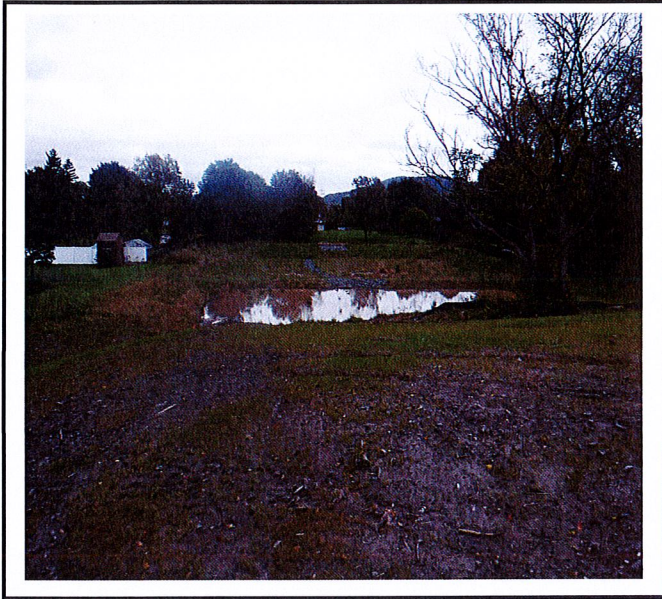
Stormwater forebay still too wet to dredge out.
