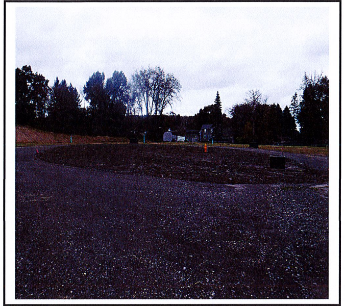
Center of island not stabilized with seed and mulch.
