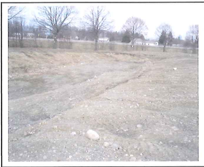
Stormwater basin rough graded.
