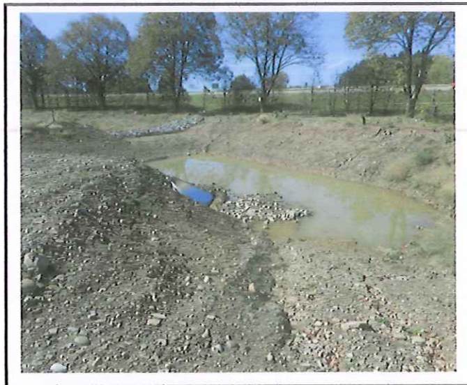
Forebay is being utilized as a sediment basin.
