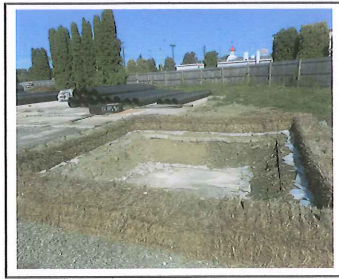
Concrete washout pit.
