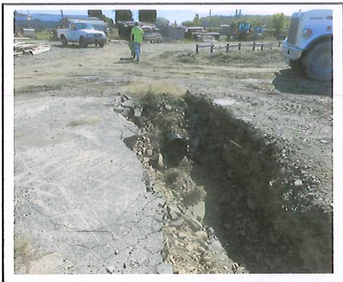
Storm sewers are partially installed.
