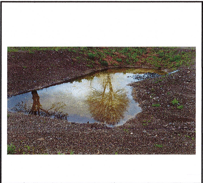
Stormwater forebay of basin.
