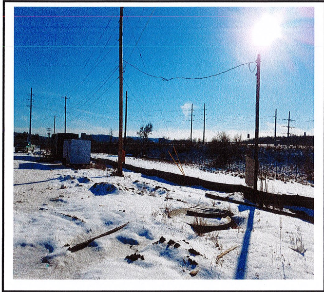
Silt fence has been replaced.
