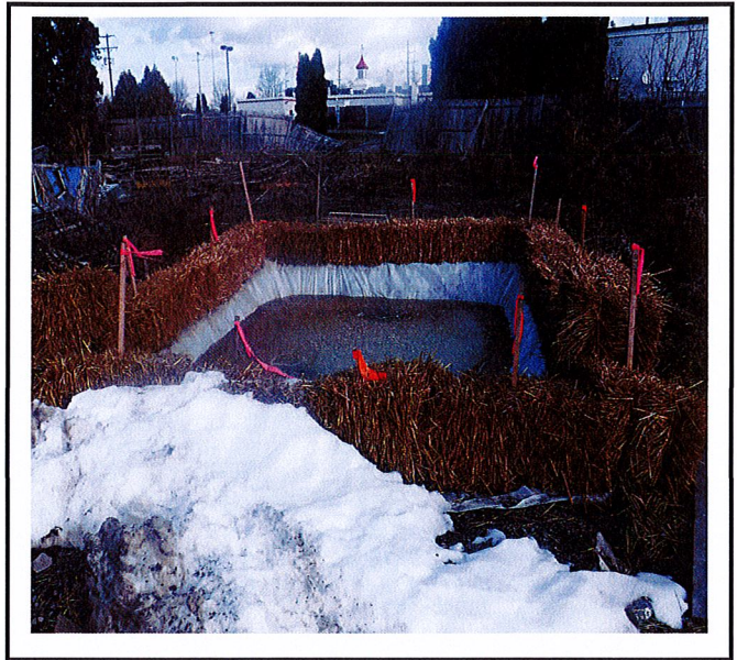
Concrete washout has been installed.
