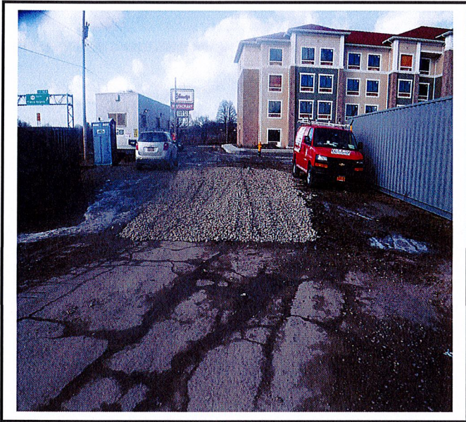
Construction entrance has been installed.
