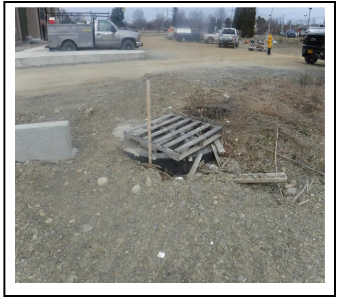
Grading is getting to the point where drop inlet protection is needed in areas where water can get into the stormwater system.
