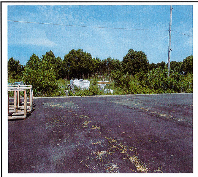
Woody vegetation growing around the stormwater basin.
