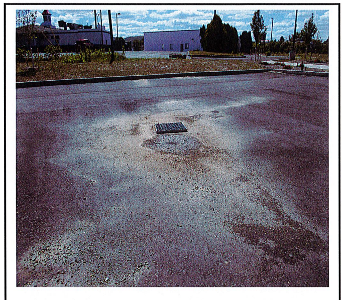
Soil around the entire site needs to be protected from erosion so that sediment doesn't get into the storm system.
