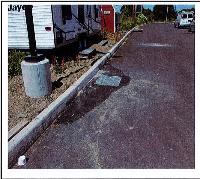
Repaired concrete curb.
