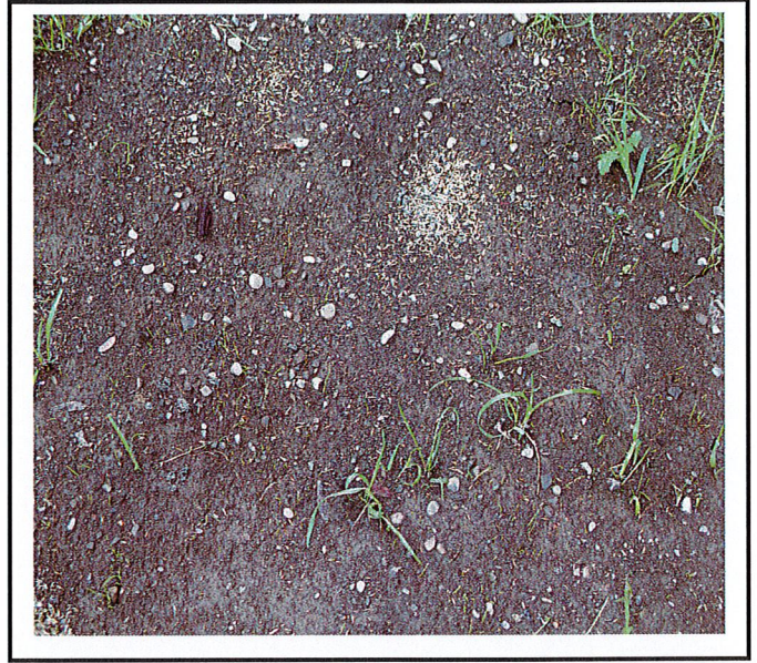
Seeding rate along south end of building will not establish 80% vegetative cover.
