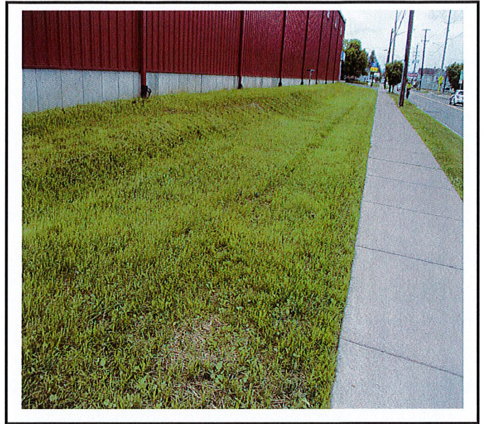
Swale along College Ave.
