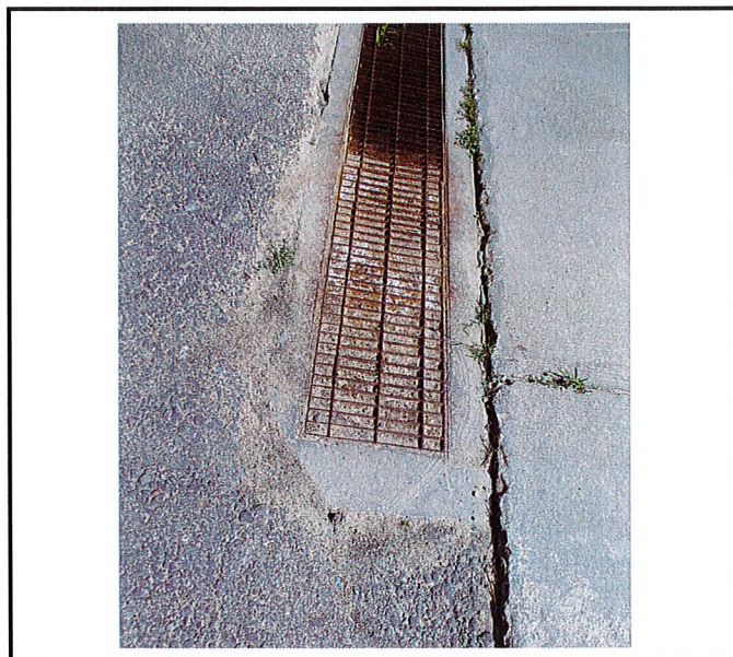
Sediment from erosion at new building has filled trench drain in parking area.
