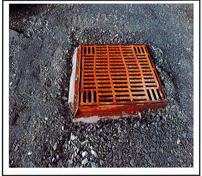
Catch basin drainage structures require protection spelled out in approved SWPPP.
