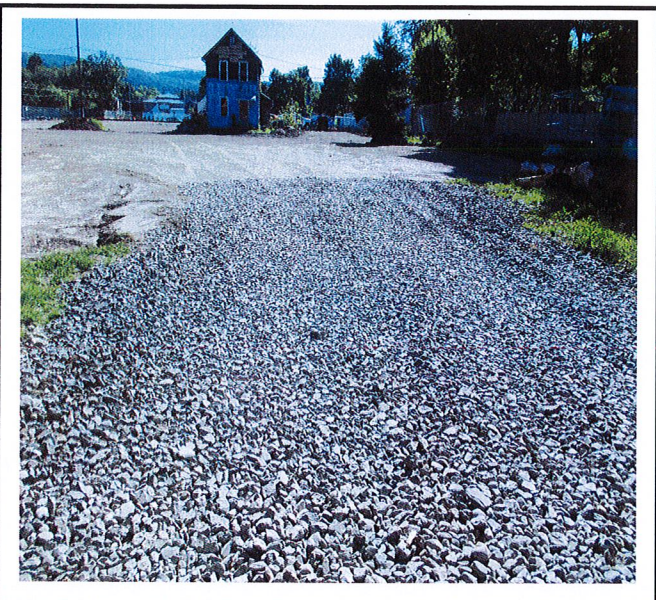
Construction entrance in good condition.
