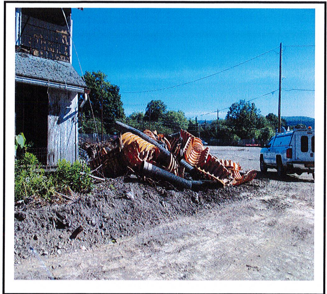
Underground infiltration from the old college parking lot has been removed.
