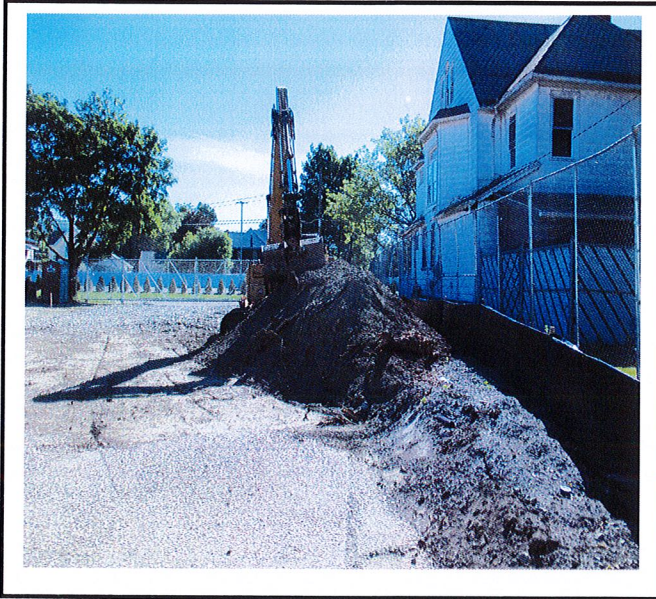
Topsoil pile is being trucked off site.
