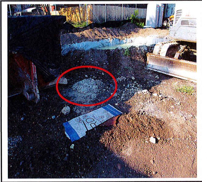
Not all concrete trucks are using the washout or getting it into the washout pit.
