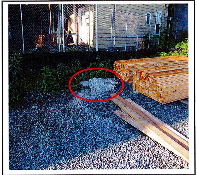
Not all concrete trucks are using the washout or getting it into the washout pit.
