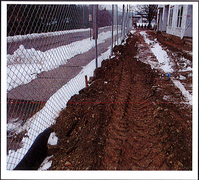
Compost sock has been buried
