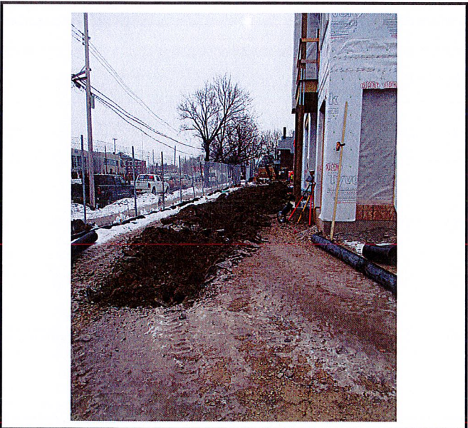
Trenches being dug for roof drainage on east side of building.
