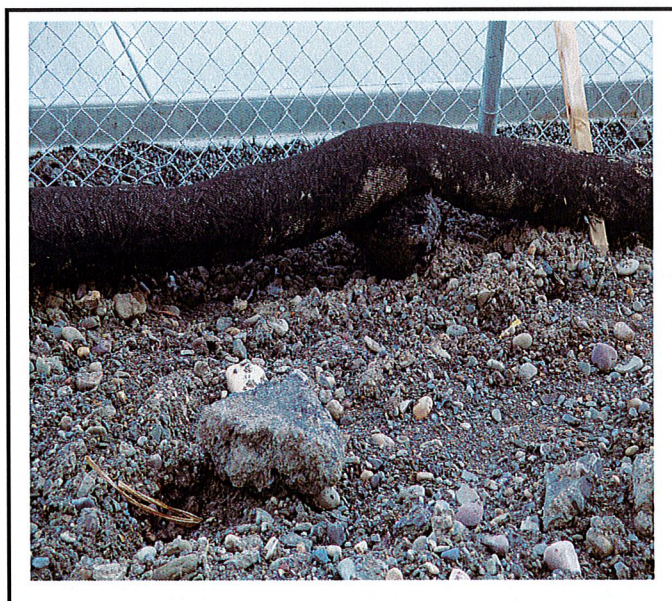
Silt sock propped up with a piece of asphalt.
