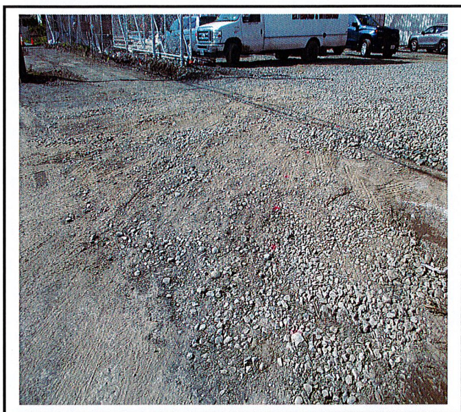
Construction entrance is in good shape but there is a lot of silt in the road. This needs to be cleaned up.
