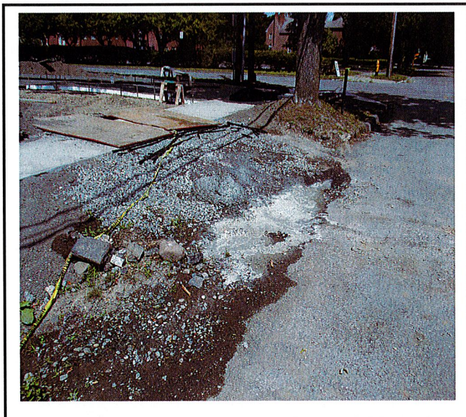
Concrete being washed directly into the road.
