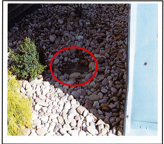
Yard drain on the west side of the building (behind porta johns) still has fabric under the grate.
