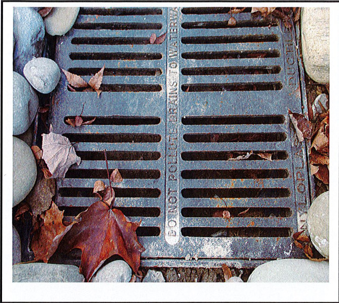
Yard drain on the west side of the building (behind porta johns) still has fabric under the grate.
