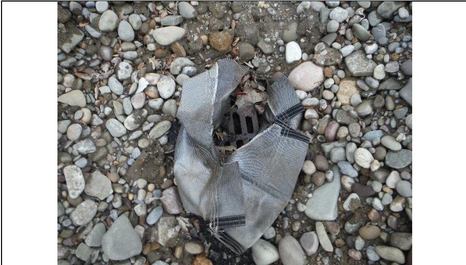
3.) Another view of storm inlet in center of property.
