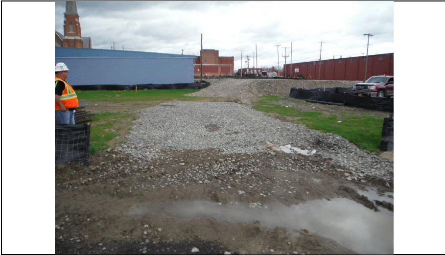
1.) Construction entrance at southwestern corner facing north.
