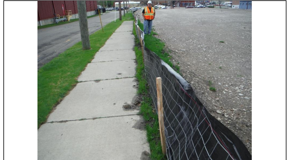
4.) Silt fence off stake. Northeastern corner of property facing south.
