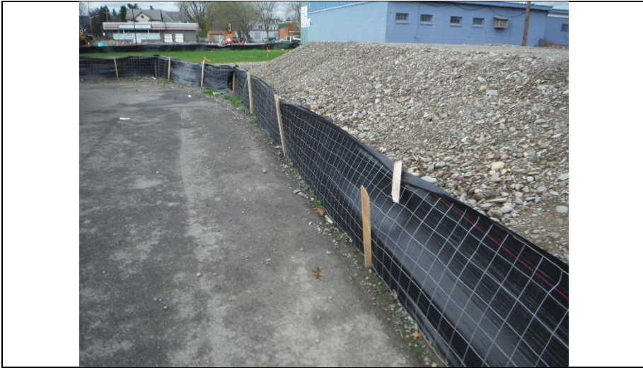
5.) Construction entrance at southwestern corner facing north.
