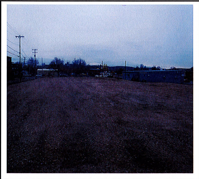
Fill material has been placed and compacted.
