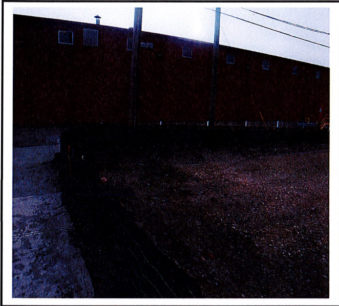
Silt fence installed.
