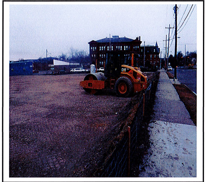
Silt fence along Clinton Street.
